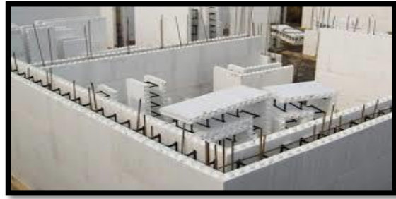
FIG 14.1.3.11 THIN JOINT MASONRY TECHNIQUE
