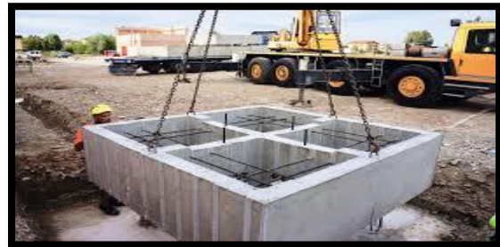
FIG 14.1.3.9 PRE-CAST FOUNDATION TECHNIQUE
