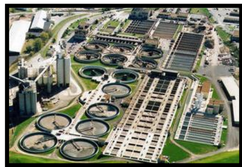
FIG 14.1.5 WATER TREATMENT PLANT
