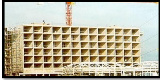
FIG 14.1.3.7 PRECAST FLAT PANEL MODULES
